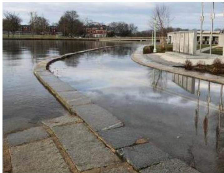
1. High tides along the curbside on the campus of the U.S. Naval Academy. Flooded more than 90 times in 2019 and 2020. (m) K/Rebel
